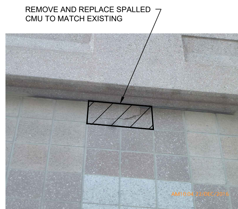
5 CMU REPAIR DETAIL NOT TO SCALE
