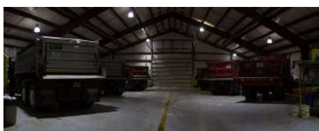
BEFORE: Pre-Existing LED Lighting
