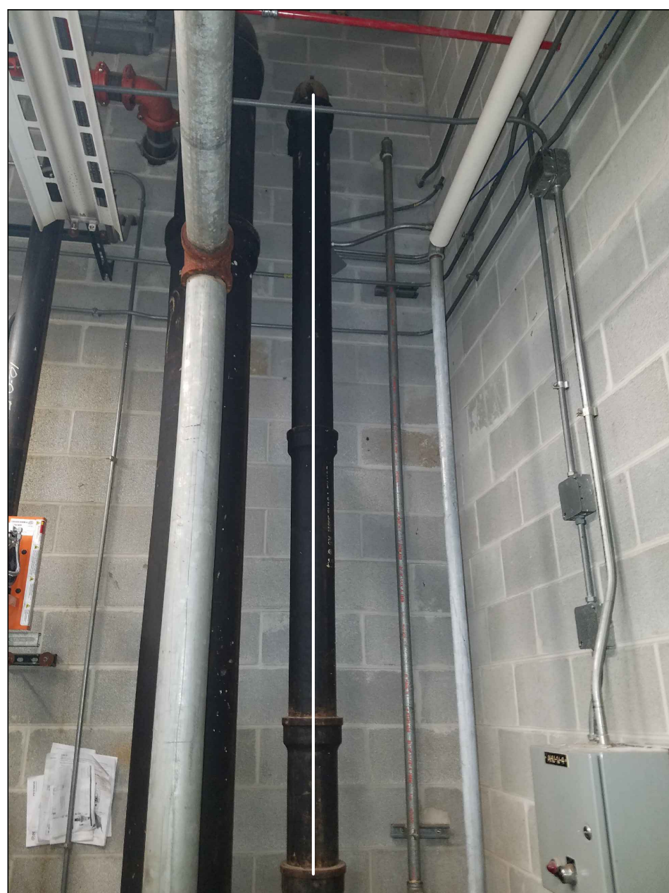
3 MECHANICAL ROOM 1.1.5 - SANITARY PIPING SCALE: NO SCALE
