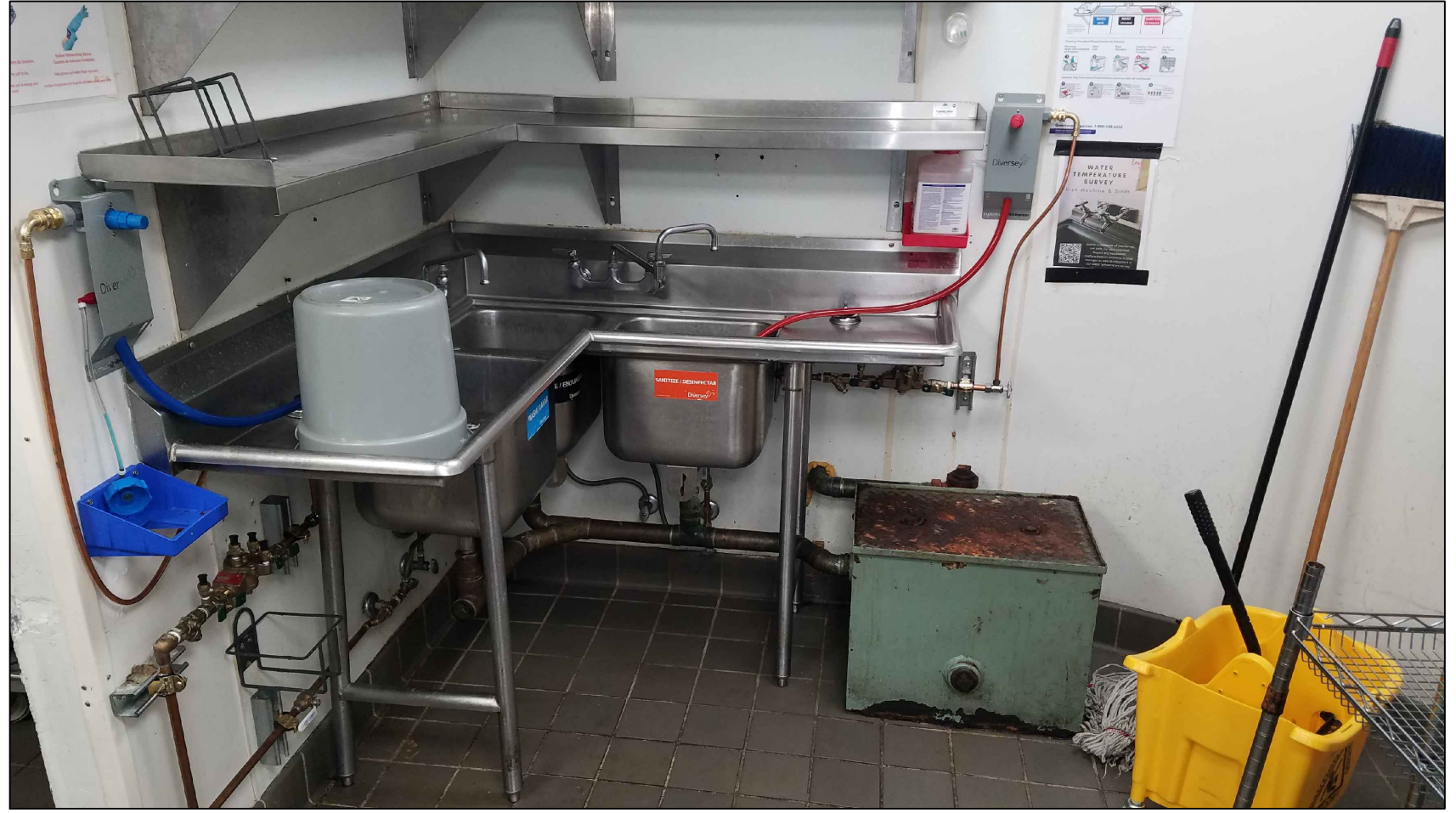
3 KITCHEN - GREASE INTERCEPTOR SCALE: NO SCALE
