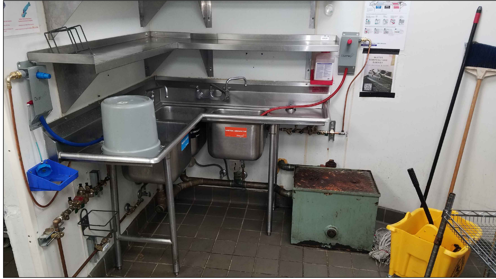
3 KITCHEN - GREASE INTERCEPTOR SCALE: NO SCALE
